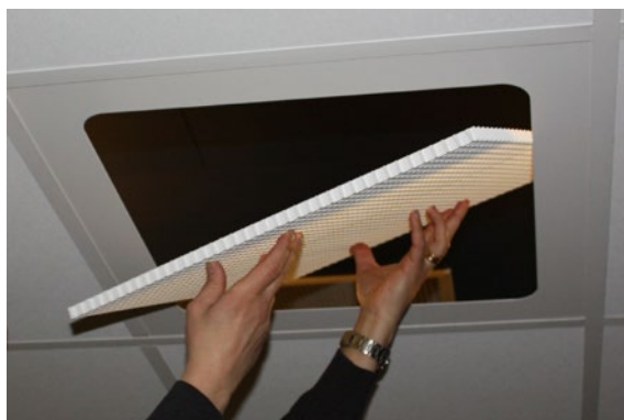
Figure 2. Raster installation in ADAPTER.
