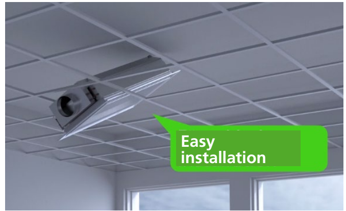
Figure 16. Installation in existing T-bar system
