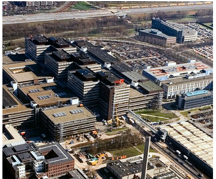
AMC Hospital - Beddenhuis, hospital, Amsterdam, The Netherlands
