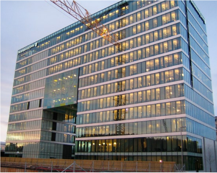
PWC, offices, Oslo, Norway
