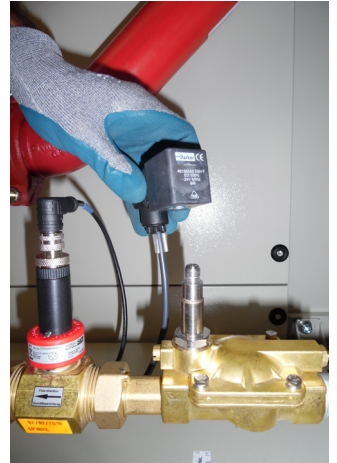
m) Pass the female connector through the lateral panel and connect it with the male one from motorized drain valve
