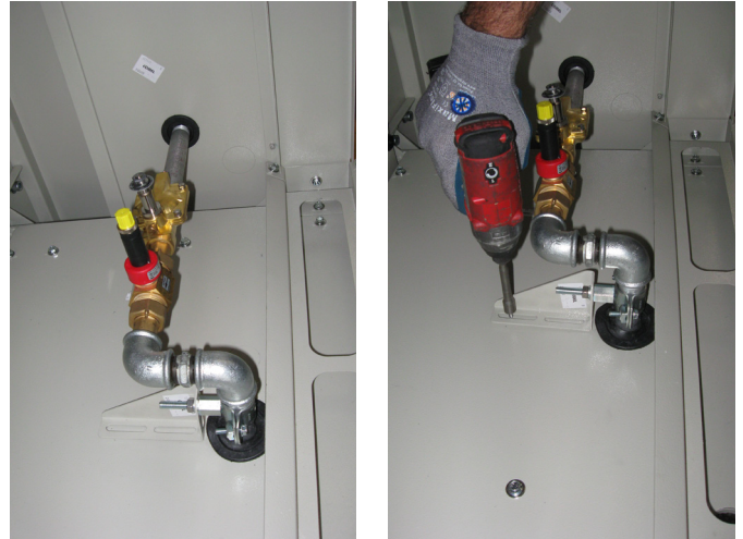
f) Mount a part of drain circuit primary tank (with bleed-off tank)
