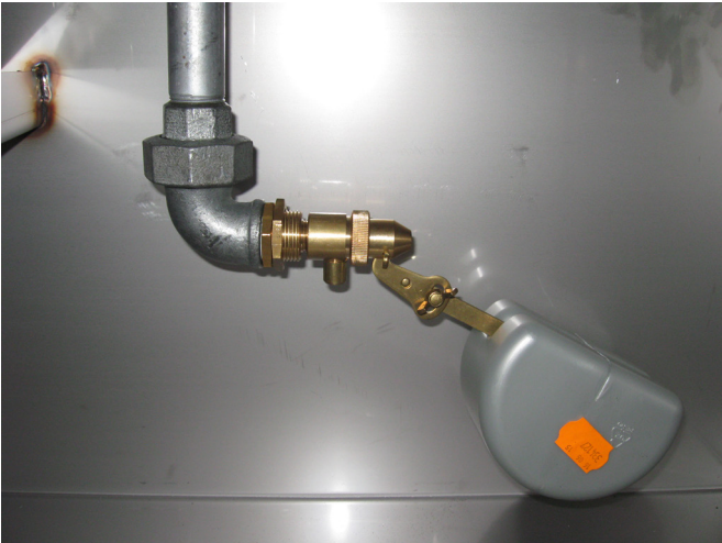
g) Mount a part of drain circuit secondary tank (without bleed-off tank)
