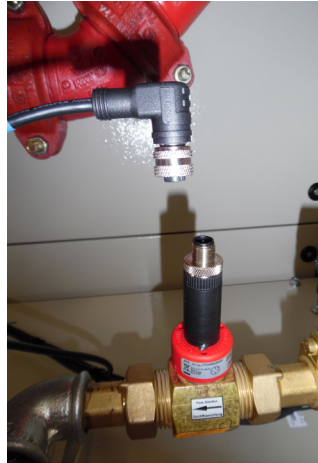
m) Pass the female connector through the lateral panel and connect it with the male one from motorized drain valve
