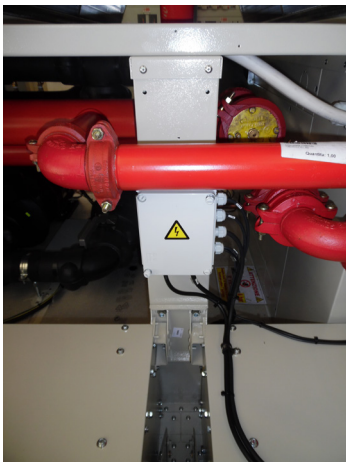
n) Open the electrical box and connect the pump and level switch
