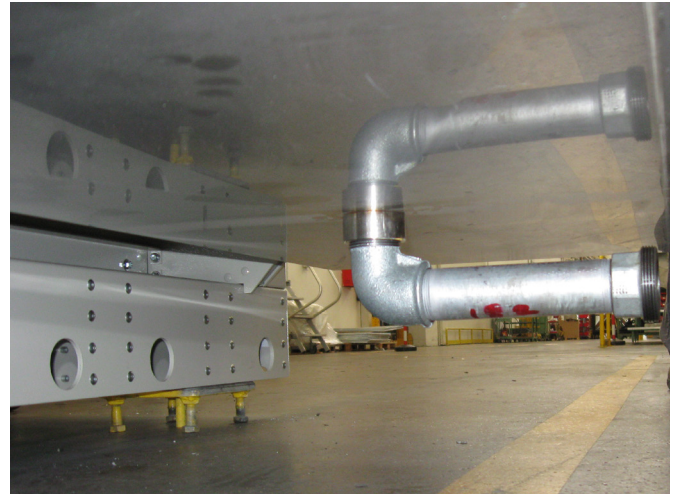
h) And connect the parts between primary and secondary by the long pipe
