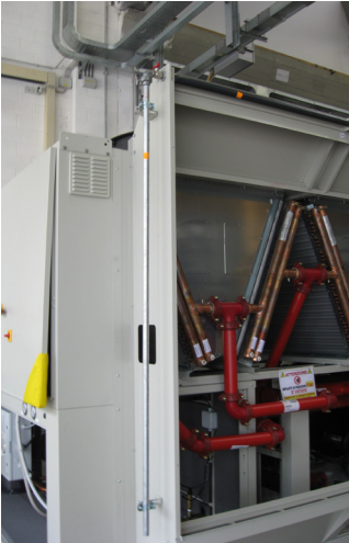
e) Mount the fill-in circuit (part 2) fixing the 3 pieces joint
