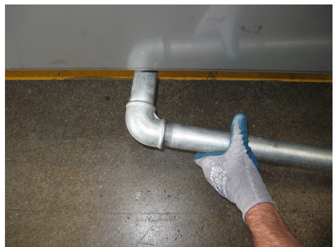
h) And connect the parts between primary and secondary by the long pipe
