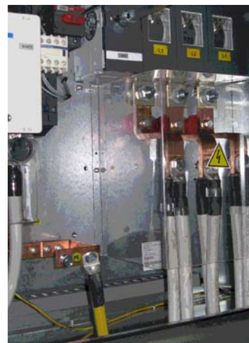
Fig. f - Restore the polycarbonate protection.
