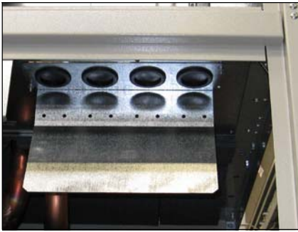
Fig. g - Restore the IP degree with cable clamps.
